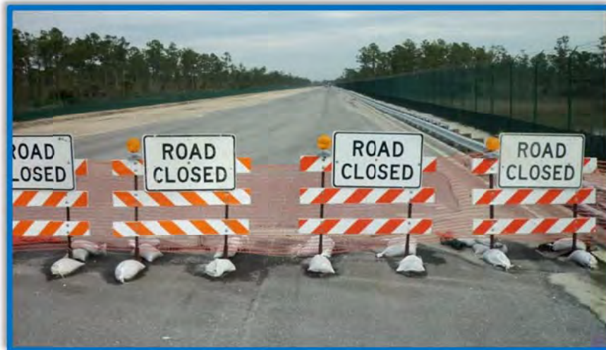
Photo: 1 – SR 7 Extension from Okeechobee Road to 60 th Street
